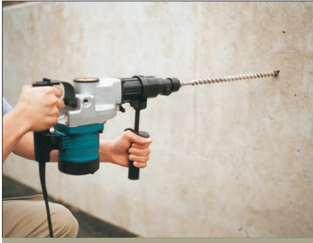
FIGURE 2-12 Hammer drill use.
