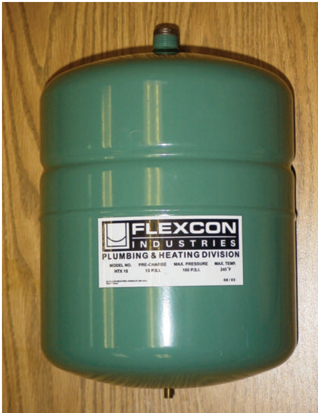
FIGURE 17–10 Steel expansion tank.
